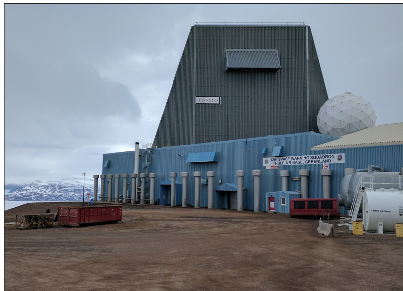
The U.S. Army Corps of Engineers upgraded the High-Altitude Electromagnetic Pulse (HEMP) shield at Bldg. 4002 at Thule Air Base, Greenland.
